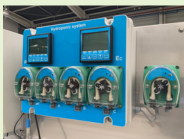
Hydroponic Irrigation (pH and EC control)
